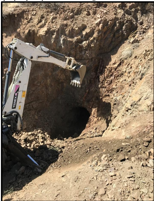
Figure 3: Backhoe exposing stope
