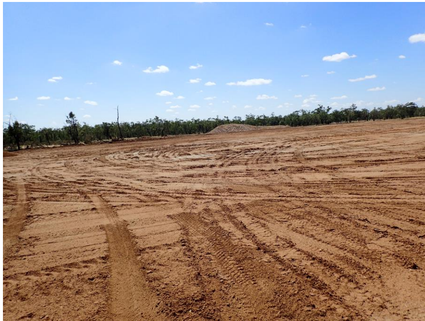
Figure 2 – Albany 1 drilling lease following construction
