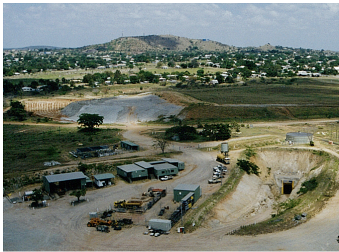
Charters Towers 'Central' mine site - Aerial view showing tunnel entrance to underground during previous operations.
