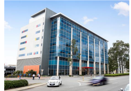
836 Wellington Street, West Perth
