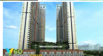
Branz, Gold Coast, West Vista Apartment Jakarta
