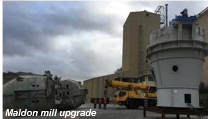
Maldon mill upgrade
