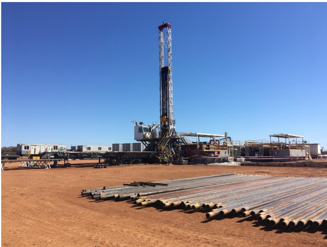
Figure 1: Ensign Rig 964 on location
