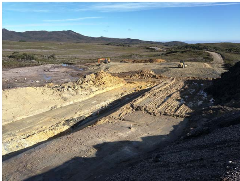
Figure 1 – Construction of northern and western embankments of the new TSF
