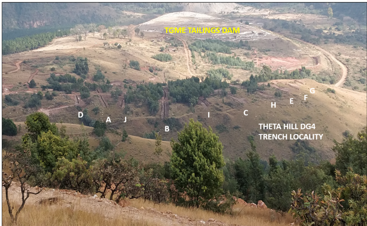
Figure 4: View showing the distribution of the trenches at DG4 (Bevetts Seam)
