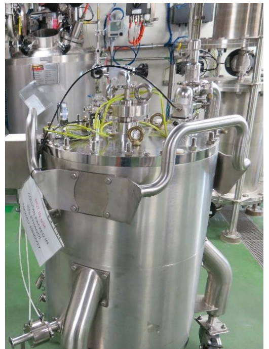
THC's Southport Manufacturing Facility (3)
