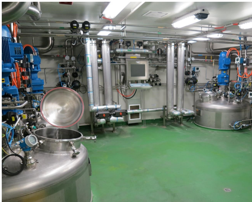
THC's Southport Manufacturing Facility (2)
