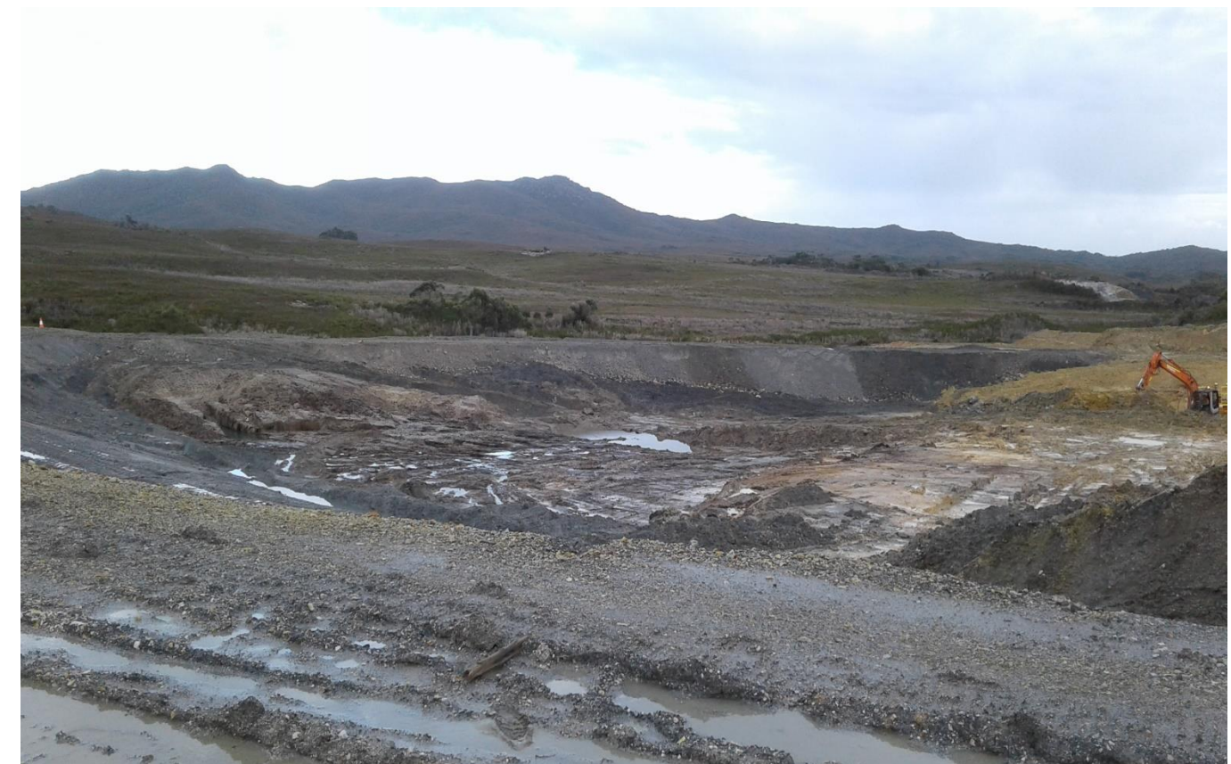
Construction of new TSF for Granville Expansion (Level 2)
