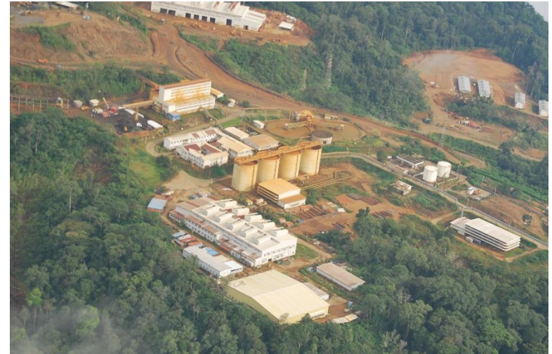
Kurumbukari mine site
