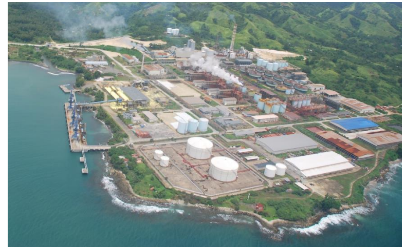
Basamuk process plant
