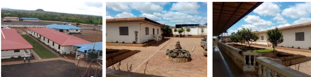
Figure 16, 17 and 18: The Luapula Processing Facility Offices and Accommodation
