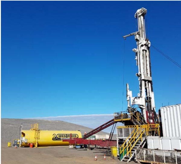
Drill rig installing Inlet Well with inlet compressor diesel tank
