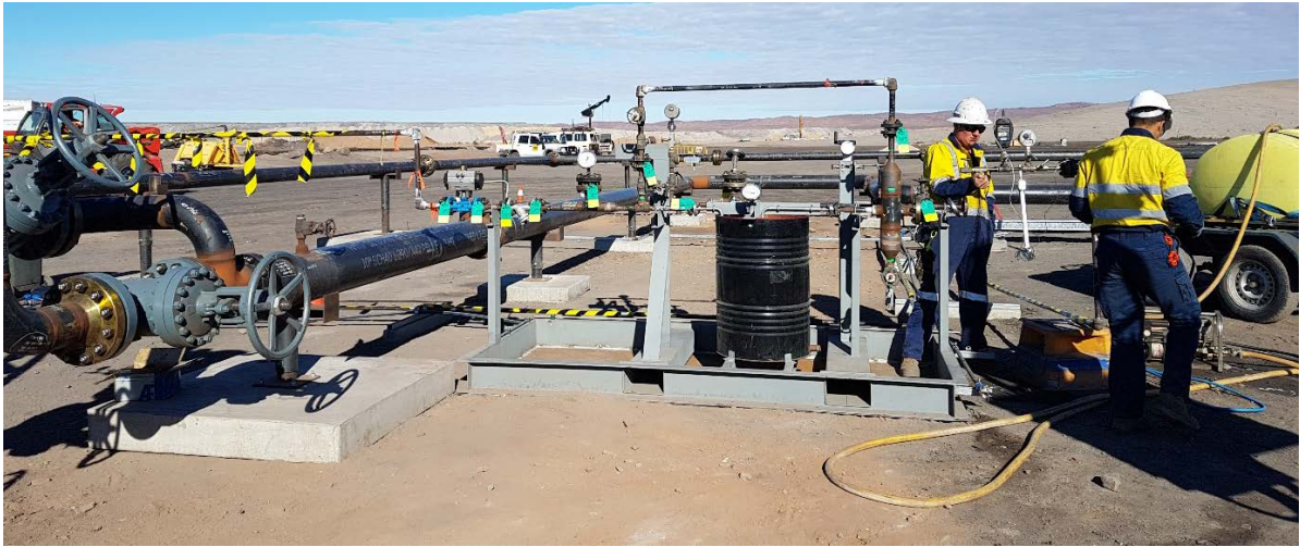
Hydraulic pressure testing of pipe infrastructure
