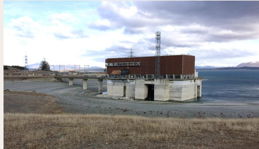
Genesis Energy's Tekapo B power station
