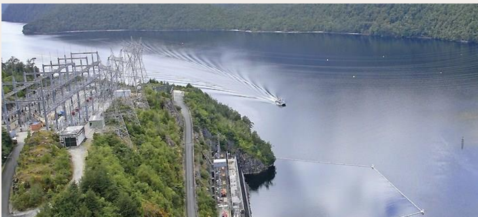
Meridian Energy's Manapouri power station
