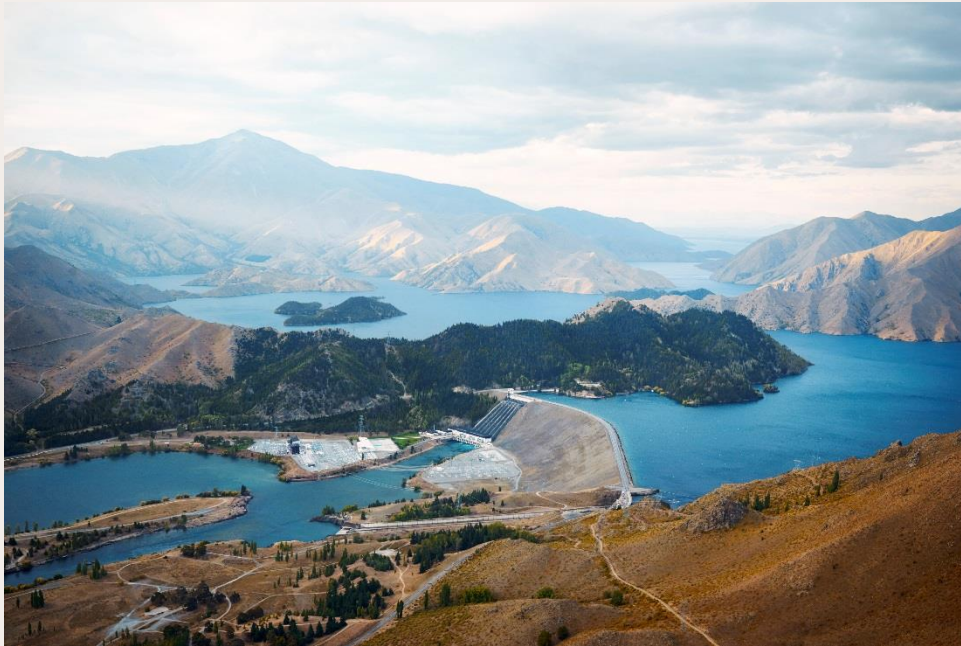
Meridian Energy's Benmore power station
