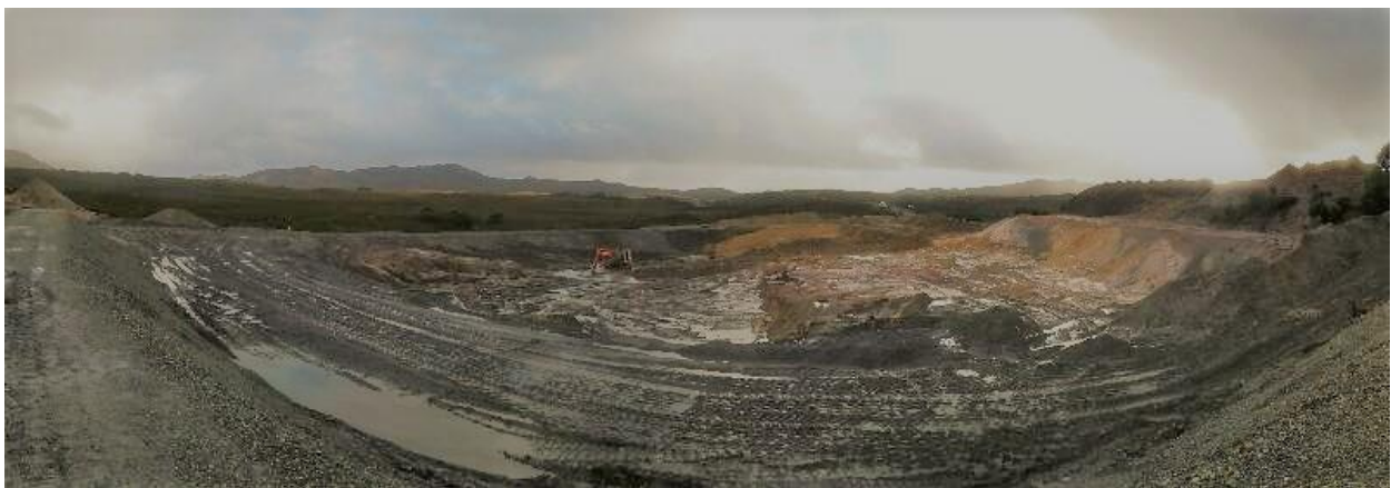
Figure 1 – New Tailings Storage Facility under construction
