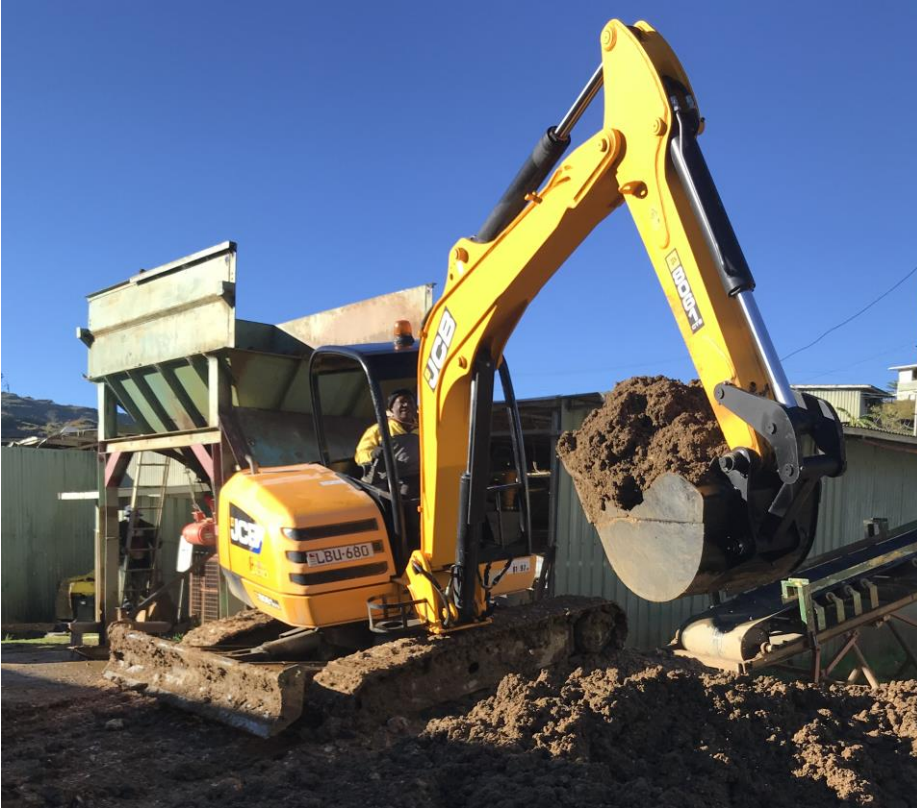
Operator Ben Tameno, loading the mill feed hopper with the new JCB excavator
