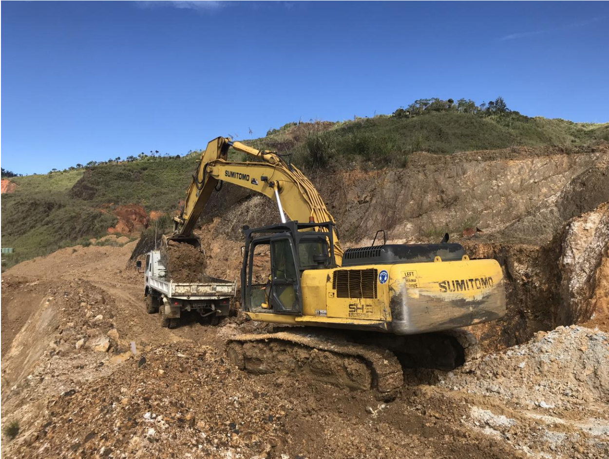
Sumitomo excavator loading vein material from the main Edie Lode at the current top bench of Alpha West
