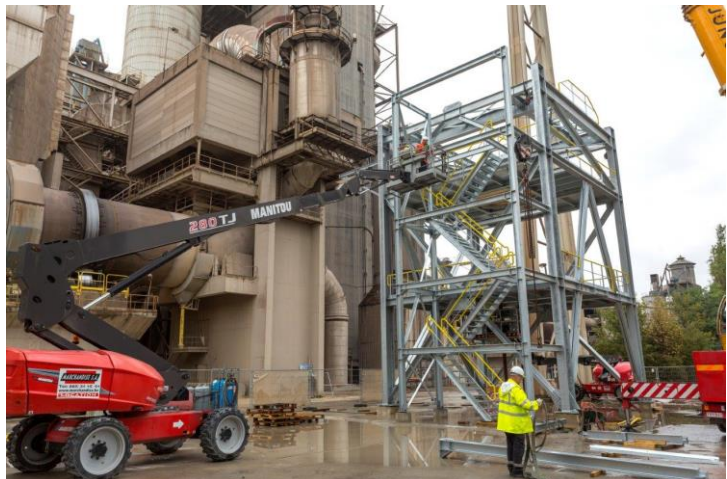
Calix's LEILAC Project – ABOVE: The LEILAC Tower construction BELOW: The LEILAC reactor bottom half being lifted into place
