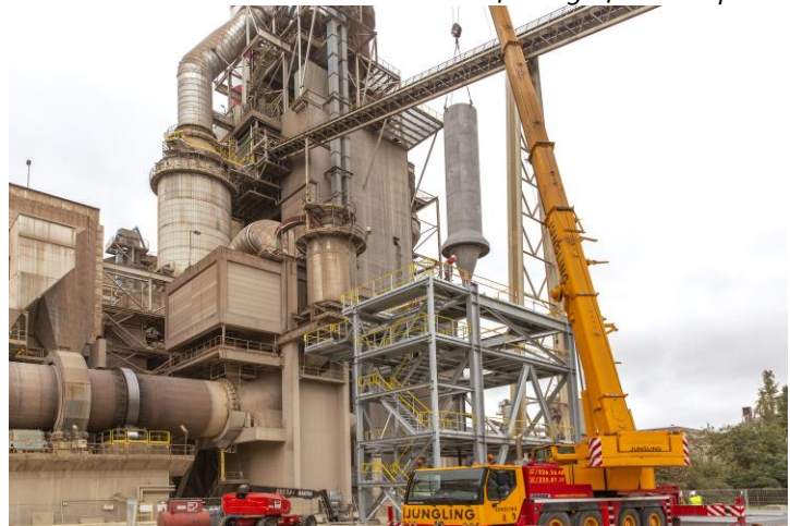
Calix's LEILAC Project – ABOVE: The LEILAC Tower construction BELOW: The LEILAC reactor bottom half being lifted into place
