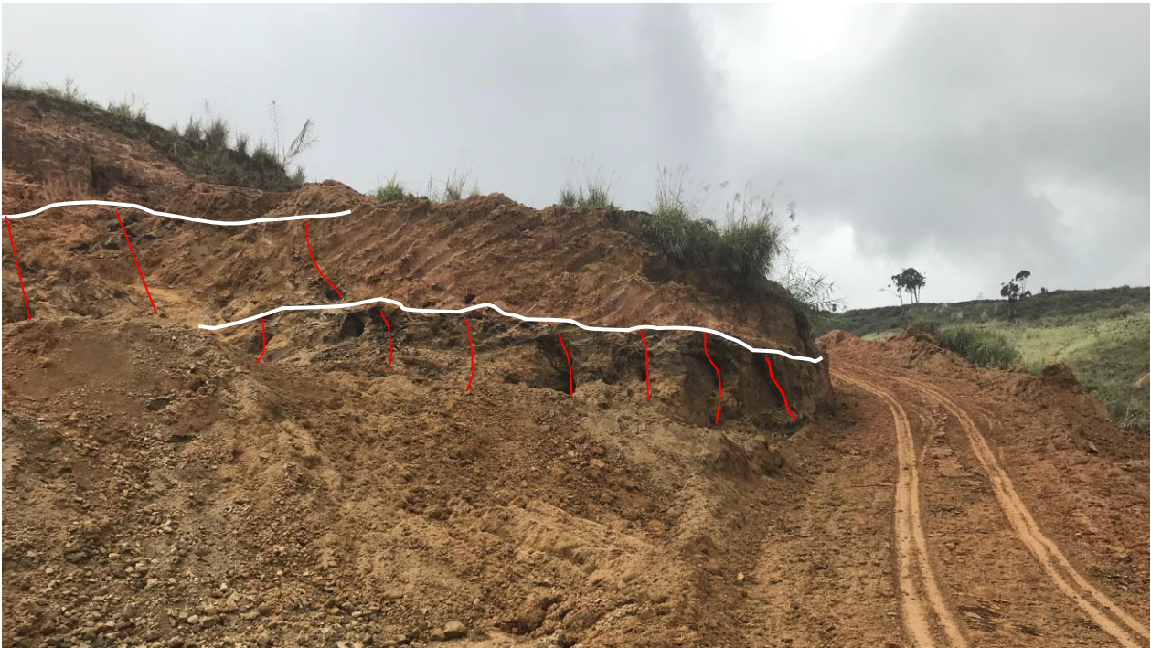
Figure 7: Shallow-dipping detachment slide fault (white line) and steeply dipping extensional faults (red lines)
