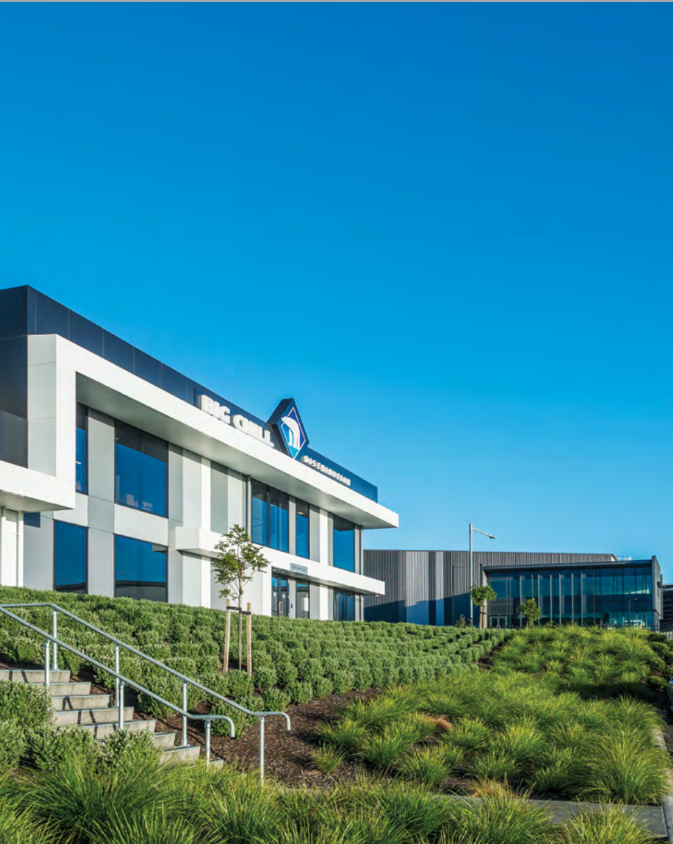
Highbrook Business Park, Auckland, New Zealand.
