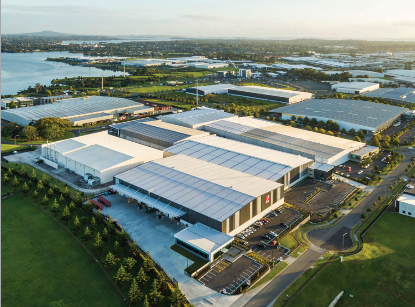
Highbrook Business Park, Auckland, New Zealand.
