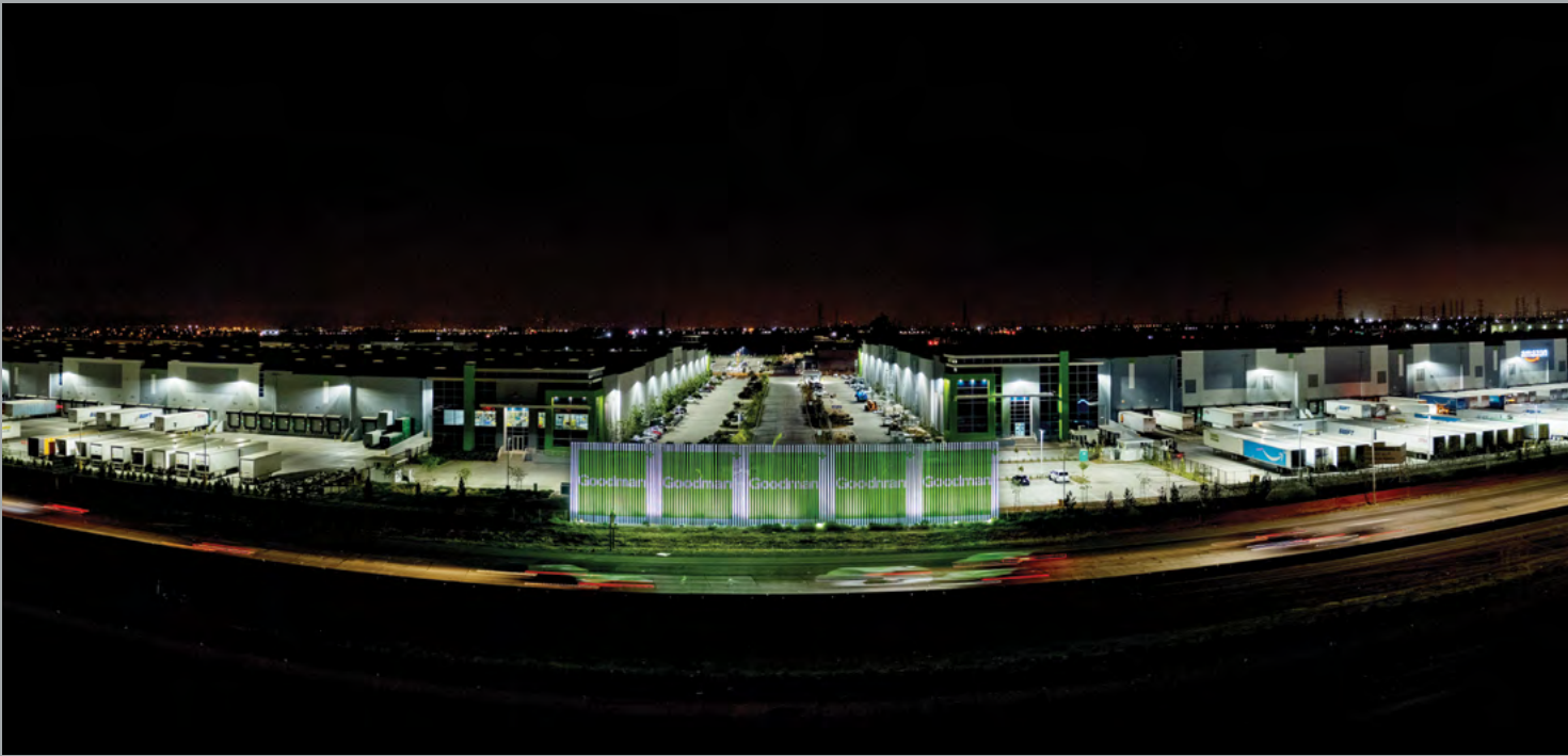
Goodman Commerce Center Eastvale, Los Angeles, USA.
