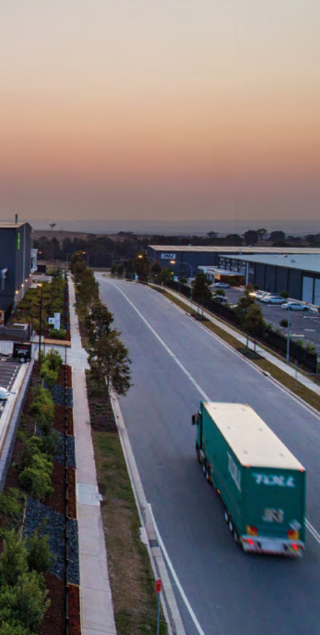
Oakdale Industrial Estate, Sydney, Australia.
