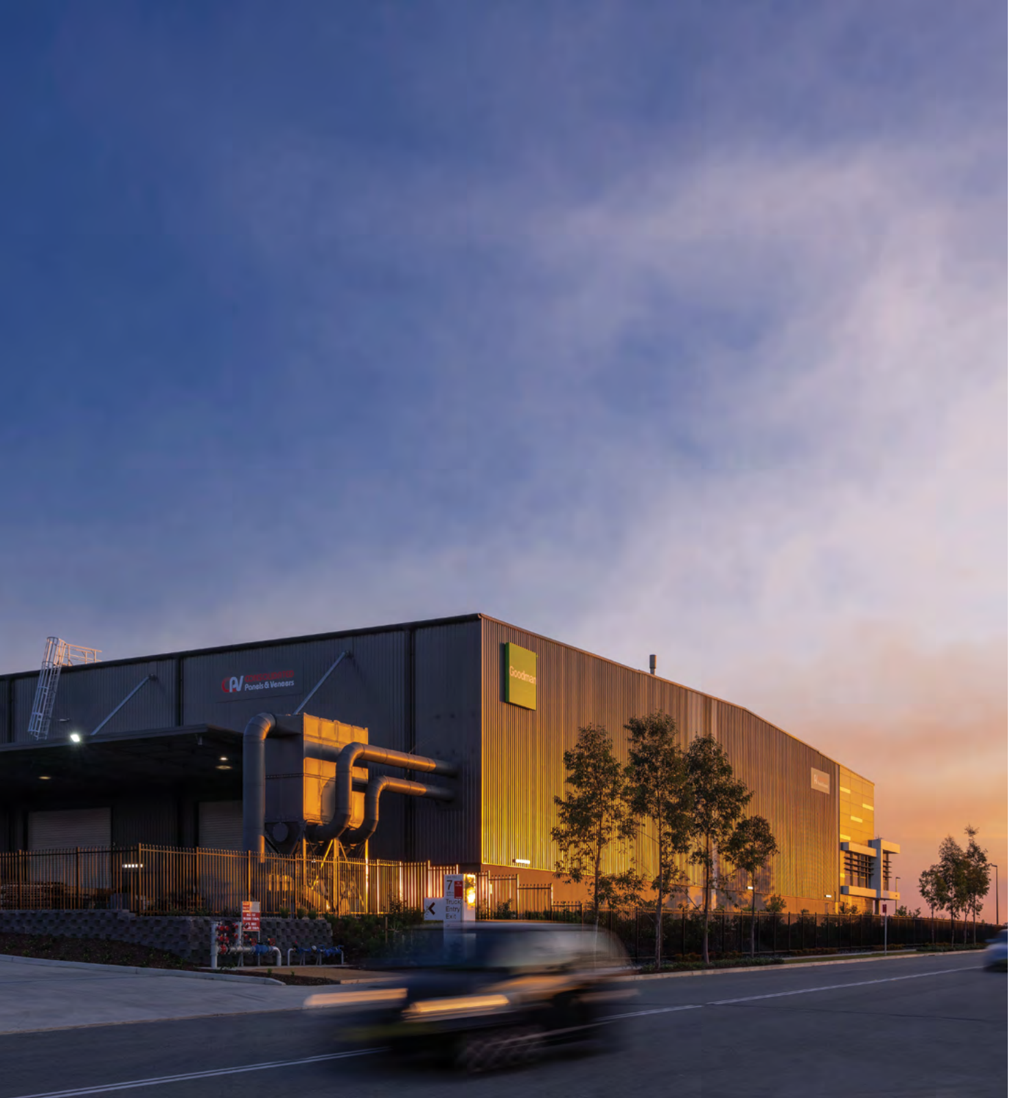
Oakdale Industrial Estate, Sydney, Australia.
