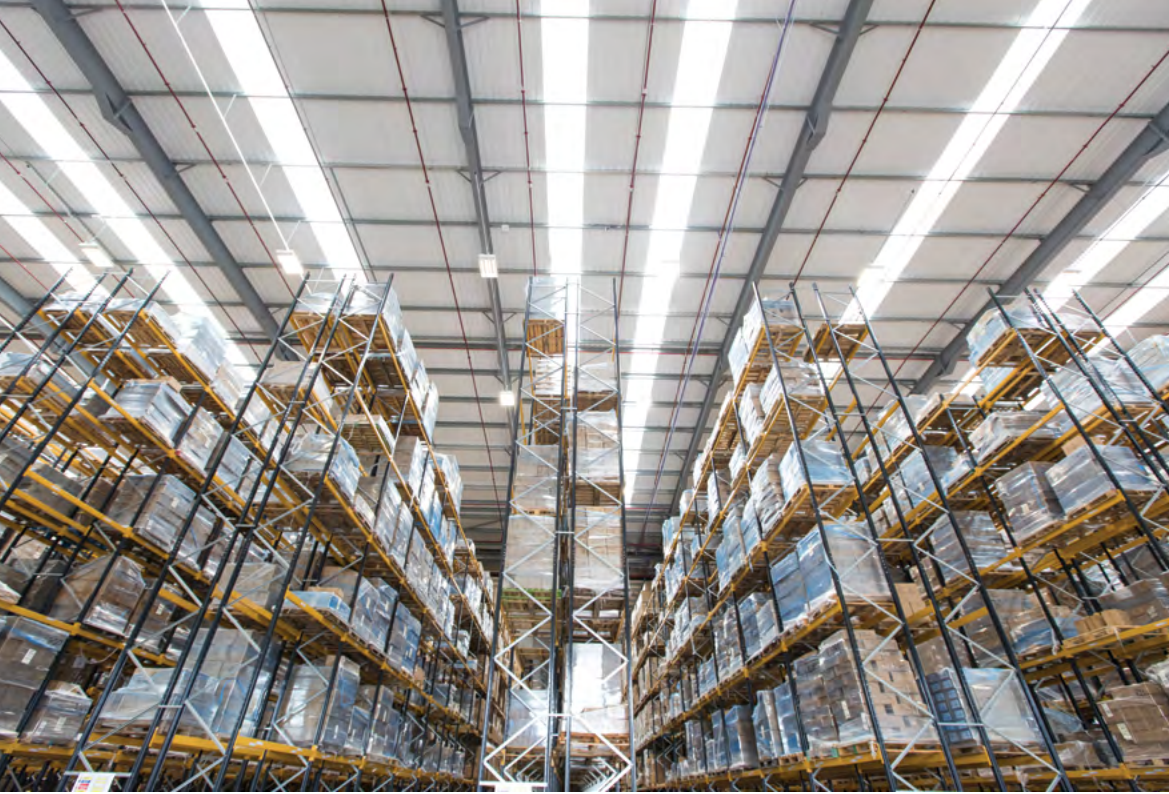
Skylights to improve natural lighting and LED lighting to improve energy efficiency.
