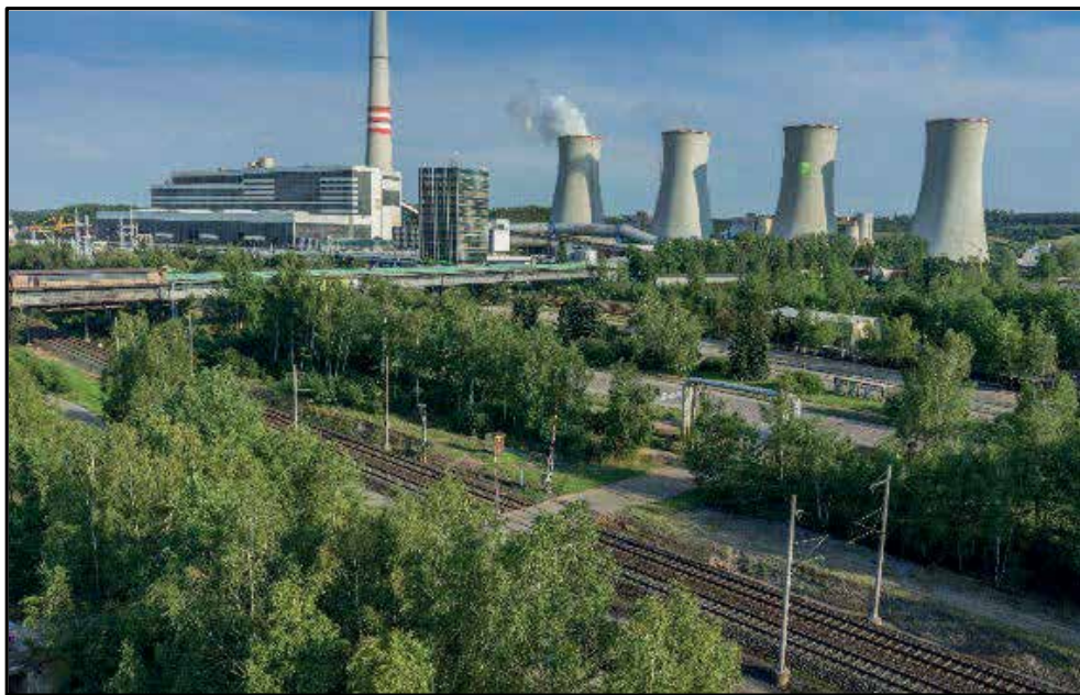
Photo 3-3: Current Power Plant
