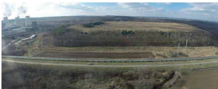
Figure 2 – Power Plant on left and tailings pile #2.
