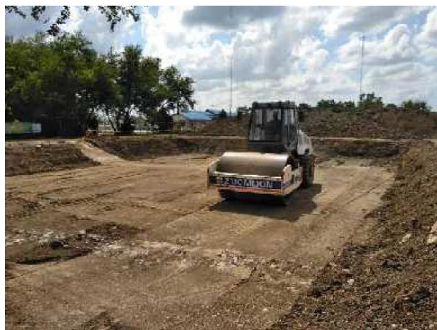
Booster compressor plinth foundations formed, compaction in progress
