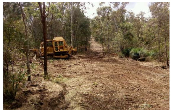
Figure 3 – Preparation of Drill Pad at Pembroke
