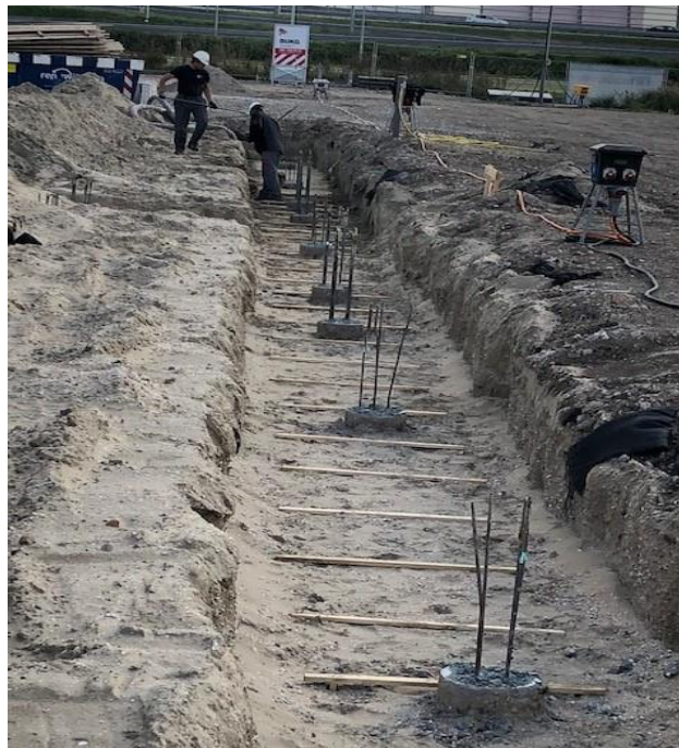
Installation of concrete slab supporting concrete beams at Amsterdam facility
