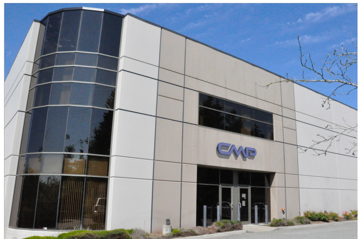
CMP's expanded facility in B.C. Canada
