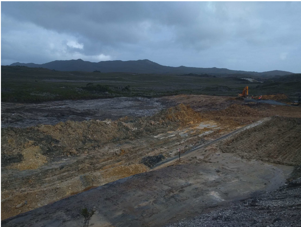
Figure 3: New Tailings Storage Facility under construction
