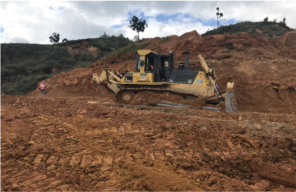
D85 bulldozer cutting a bench near the top of the Surmans vein system
