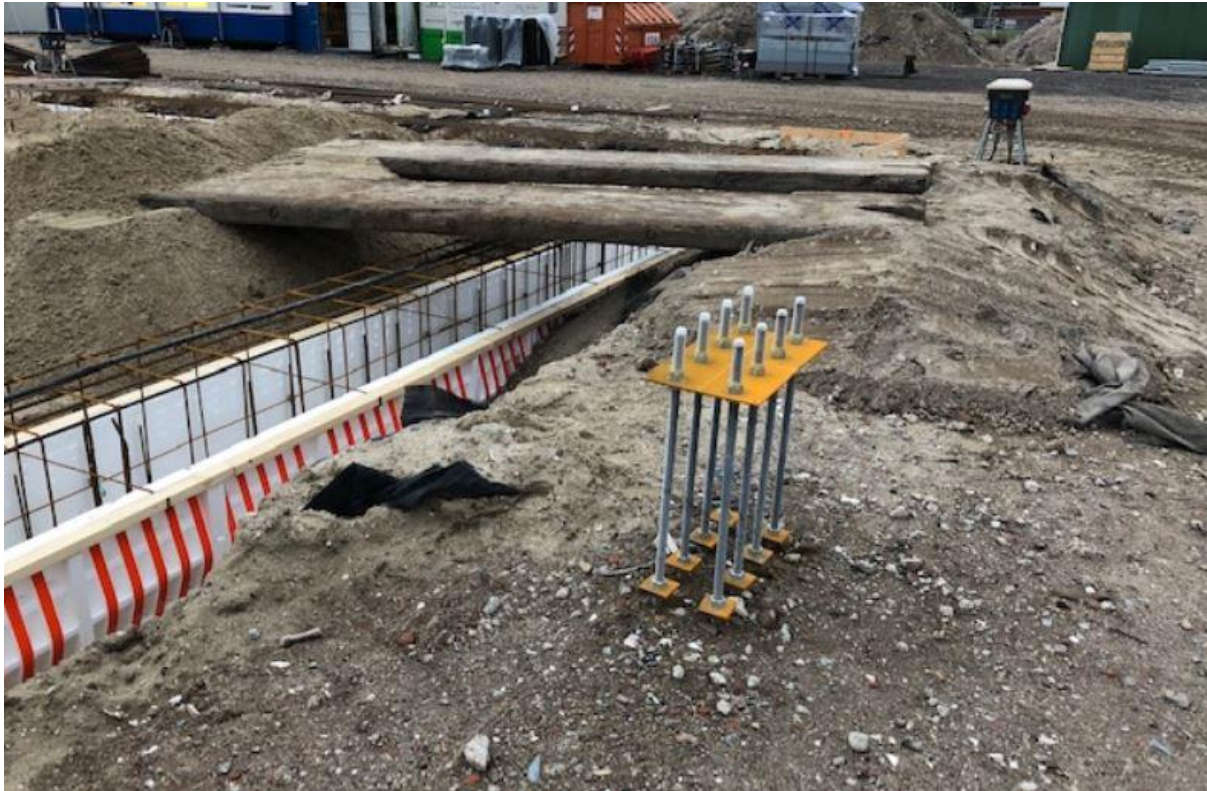
Trench to be filled with concrete, which will support the IGES fuel production building
