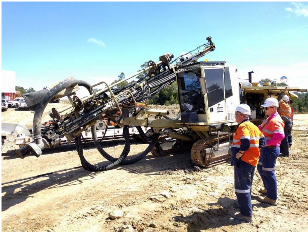
Figure 1 – Atlas Copco blast hole (production) drill recently deployed to Granville East Mine
