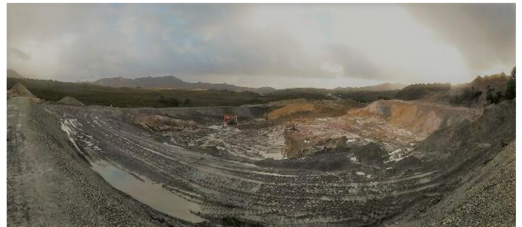
New Tailings Storage Facility under construction
