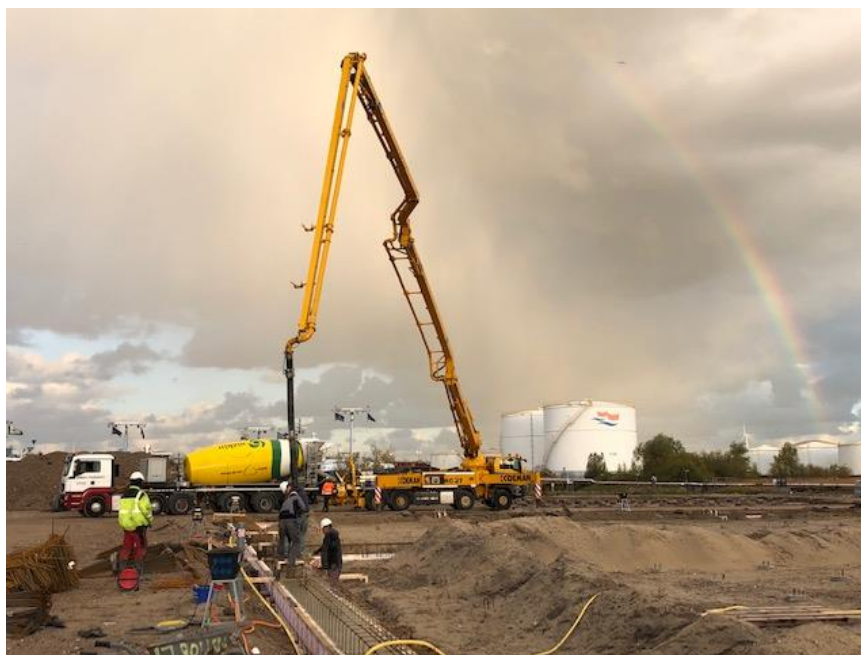
Photo of Amsterdam site showing concreting of reinforced trenches.
