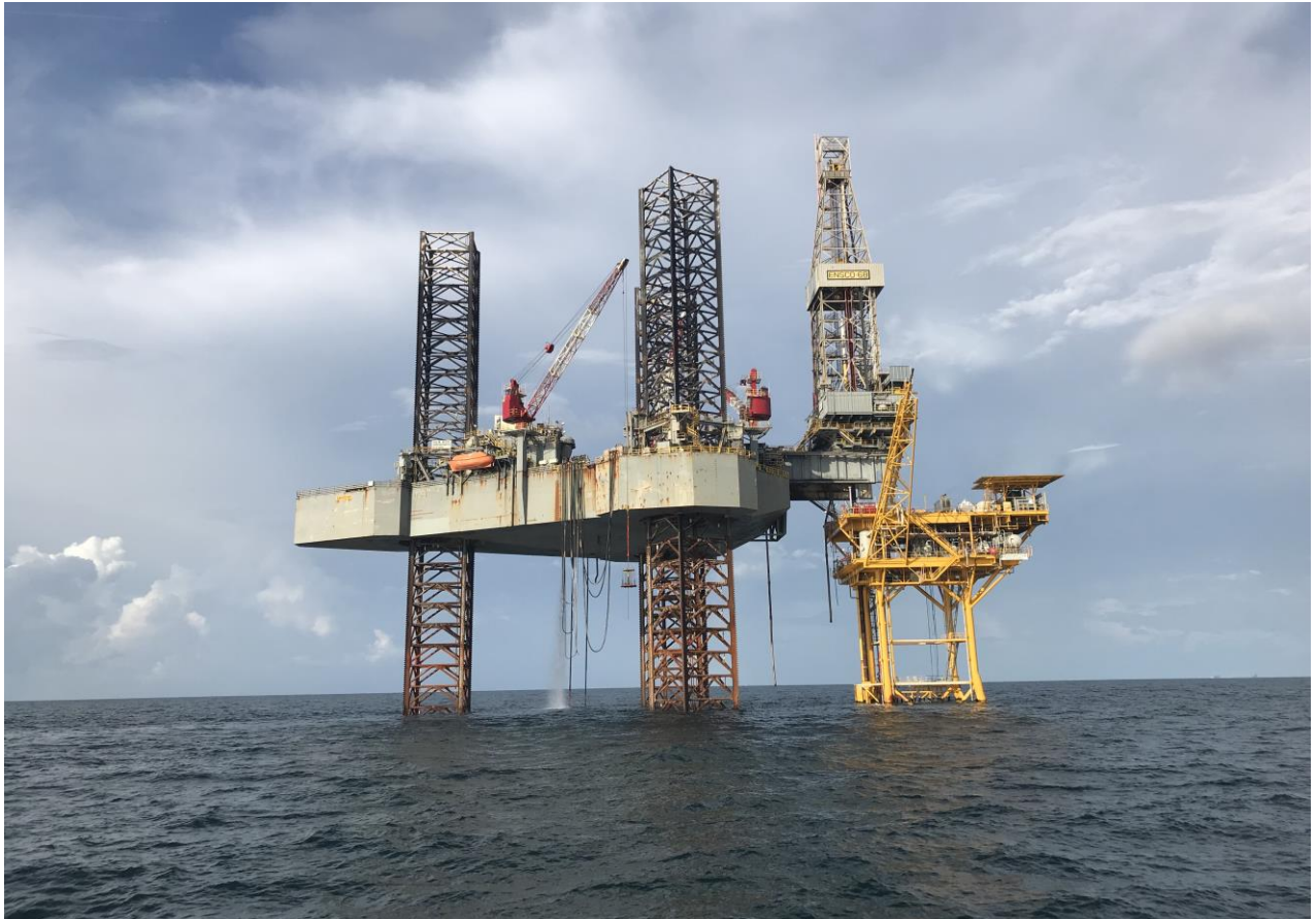
Main Pass Block 270/273/274 Hummer Project: ENSCO 68 Jackup Drill Rig
