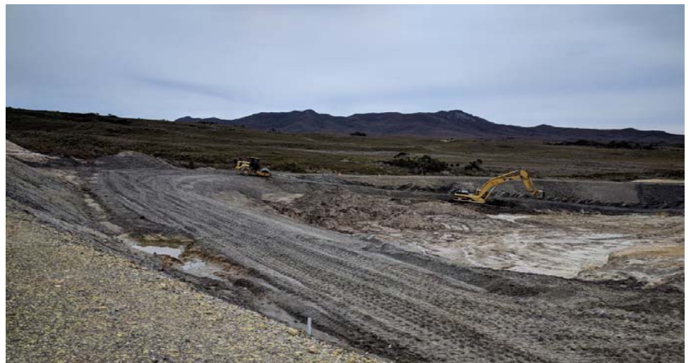
New Tailings Storage Facility under construction
