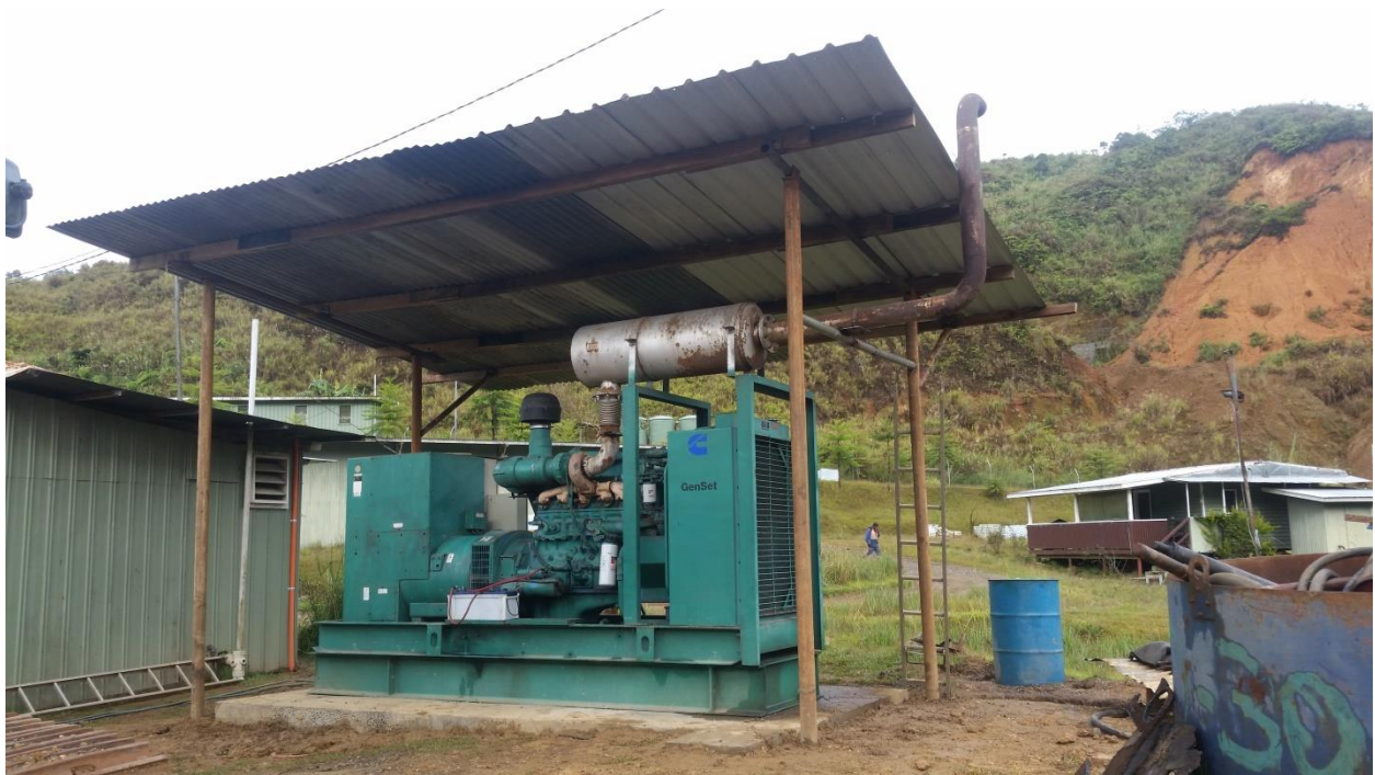
440kVA Cummins Genset installed during the year
