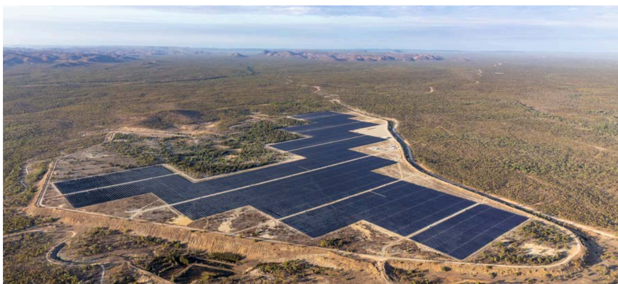
Figure 1: 50MW Kidston Solar Project
