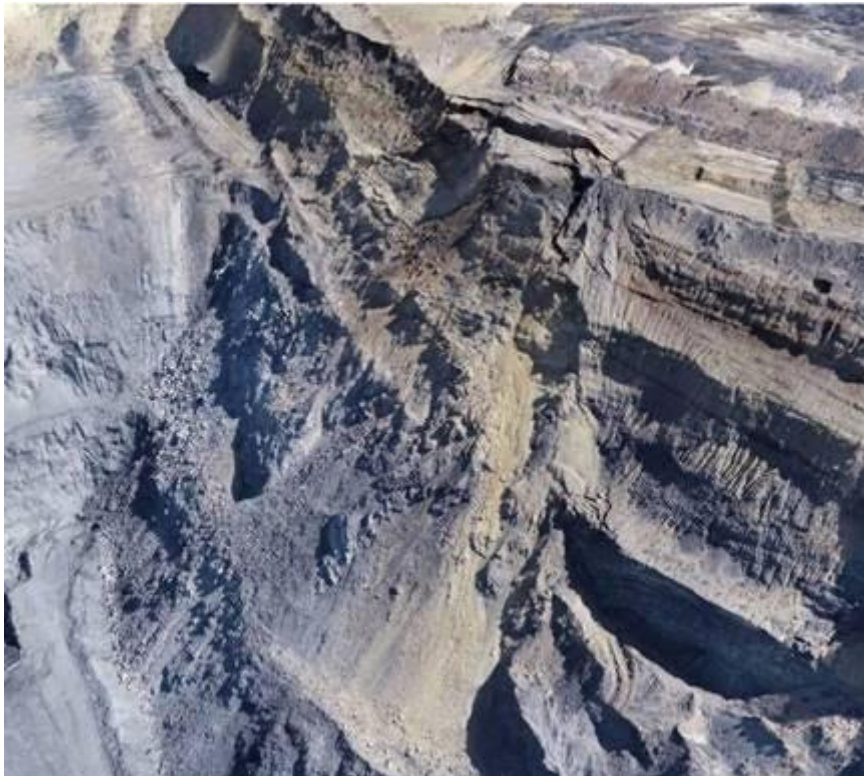
Figure 19: One Tree West Eastern End Wall Failure (14 November 2018)
