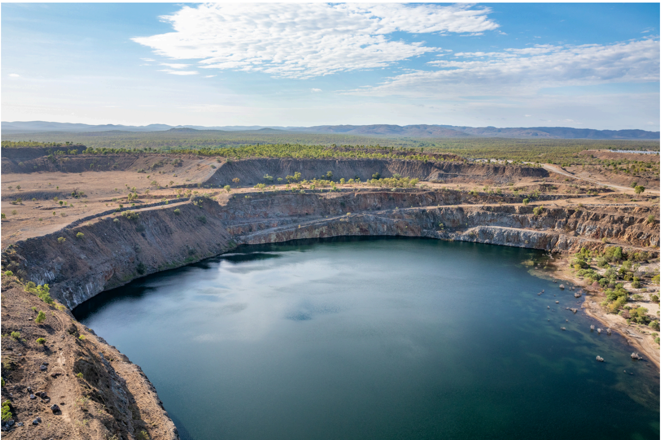
Figure 2. K2-Hydro project site – Wises Pit.
