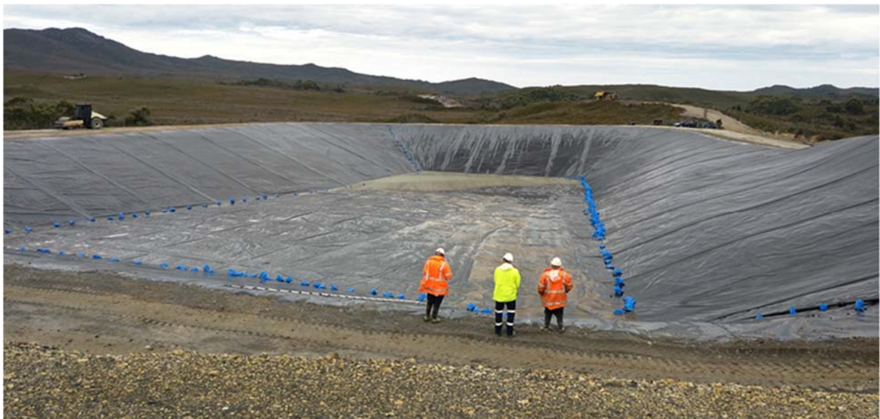
Figure 1 – New Tailings Storage Facility (TSF) at Granville Tin Project
