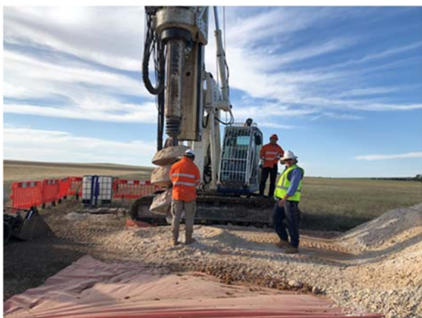
Figure 3 – Drill Rig used for Bulk Sampling Program
