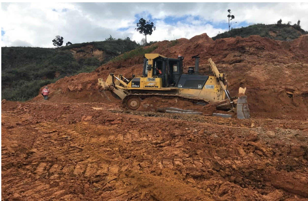
D85 bulldozer cutting a bench near the top of the Surmans vein system
