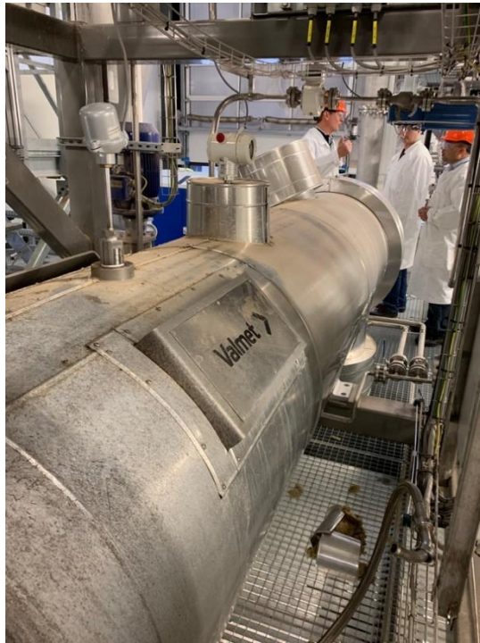
Primary pretreatment reaction in the pretreatment reactor vessel at BPF.
