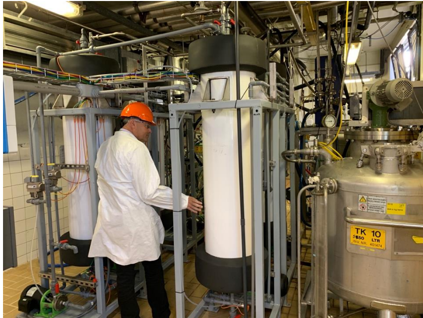
C5 sugar/glycerol separation with simulated moving bed Chromatography (SMB) unit installed at BPF.
