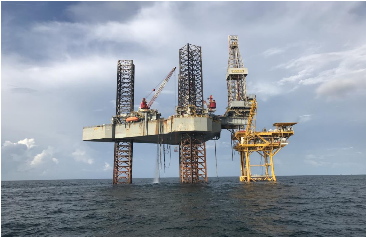
Main Pass Block 270/273/274 Hummer Project: ENSCO 68 Jackup Drill Rig
