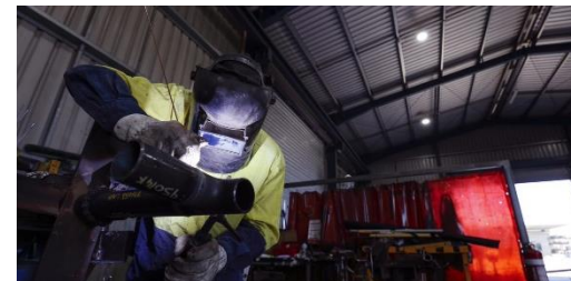
Welding during Roma North construction
