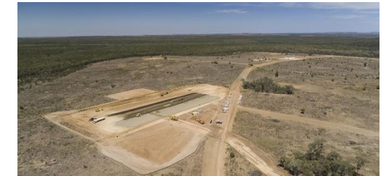
Roma North gas facility pad
