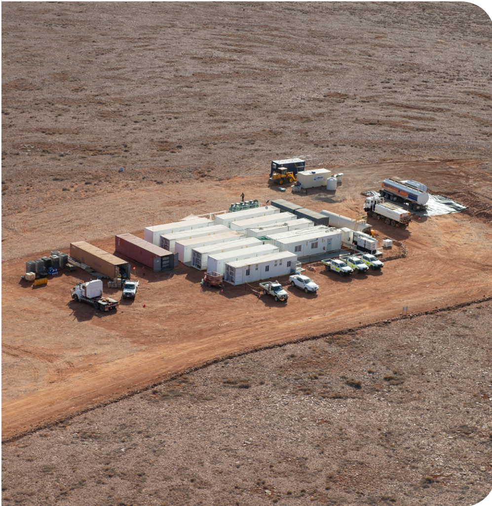
21 person camp to support 24/7 drilling
