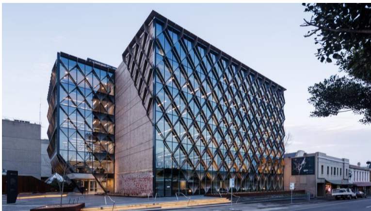
Barwon Water, Geelong VIC, featuring Capral Curtain Wall 175
