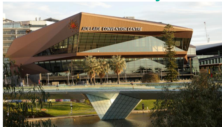
Adelaide Convention Centre SA featuring Capral Commercial Framing
