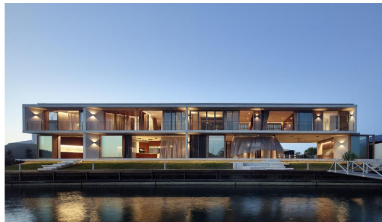
Moololah House, Brisbane, featuring Amplimesh Supascreen security sliding doors and fixed panels
