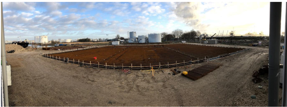
Site overview of full production plant (production area and feedstock area)
