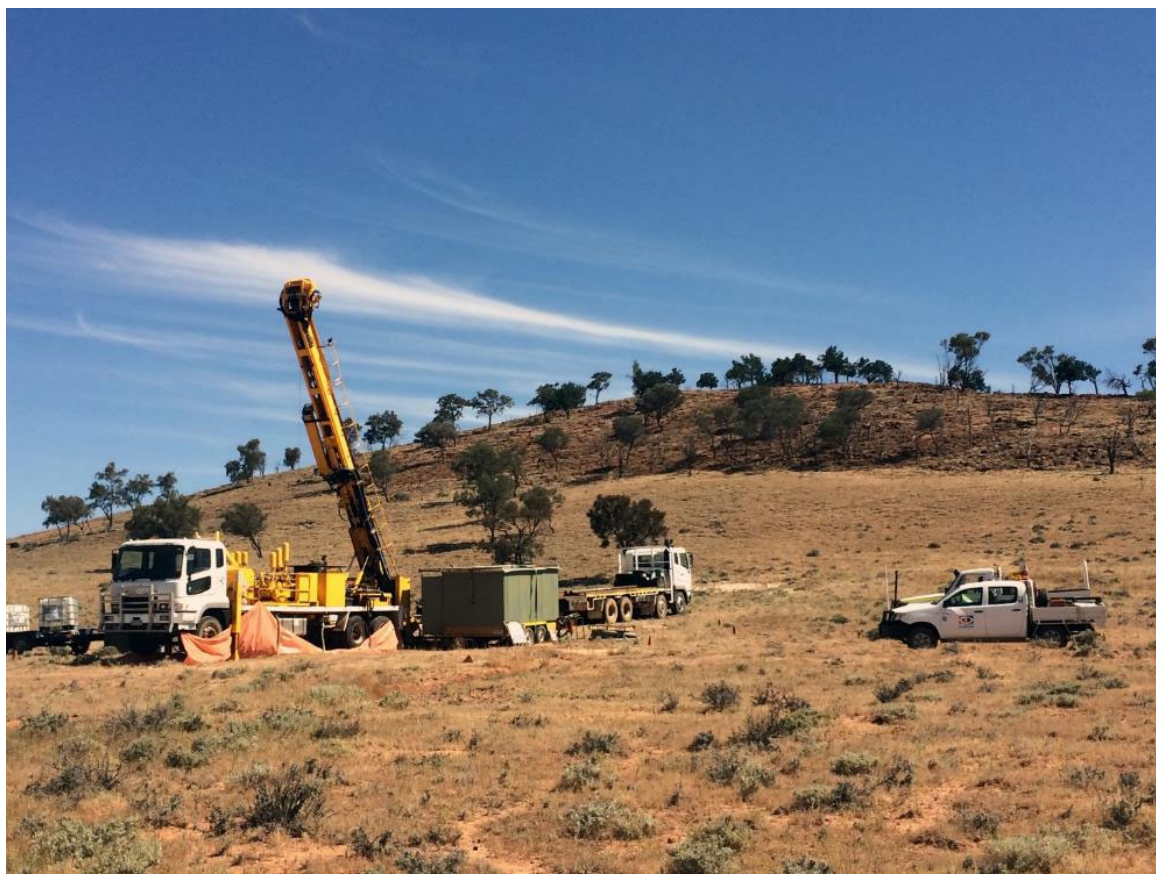
Photograph: Drilling at Thackaringa Cobalt Project
