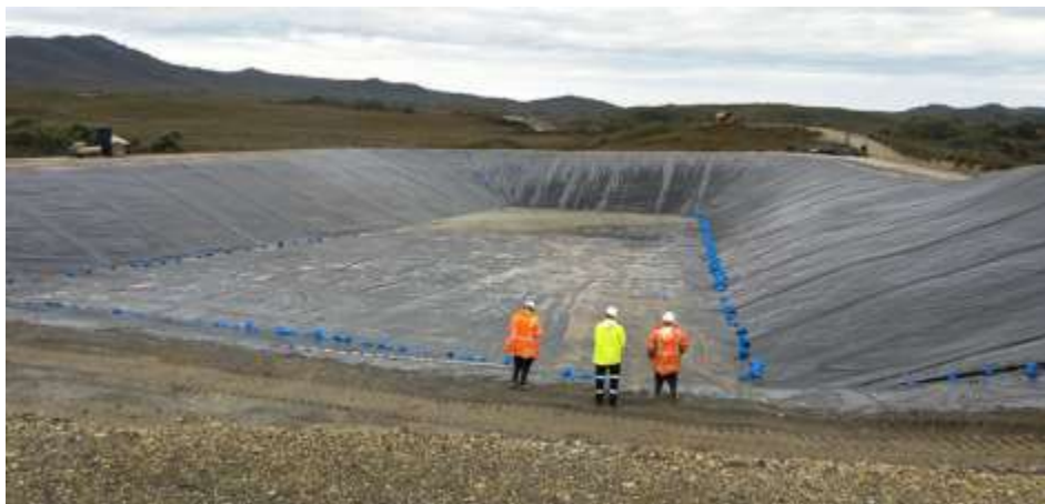
Figure 2 – New Tailings Storage Facility (TSF) at Granville Tin Project
