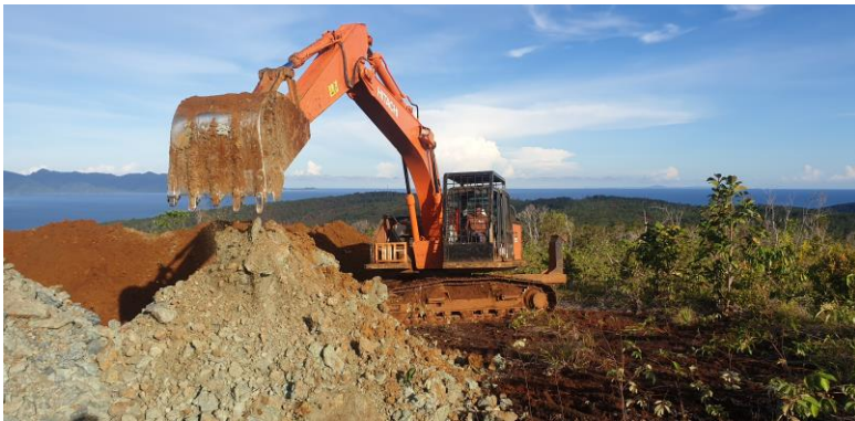
Excavation of Ni bearing Saprolite from recently opened pit
