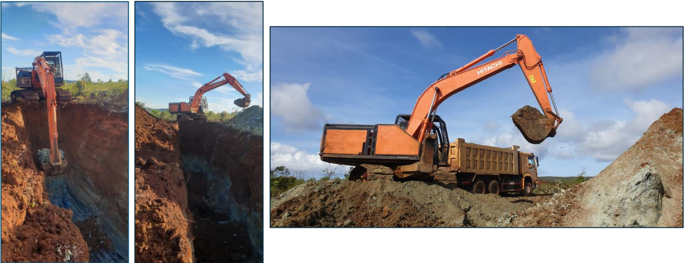
Excavation of pit II with 3m of overlying high Fe limonite with basement saprolite
