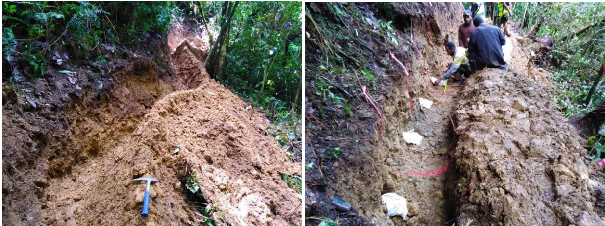
Figure 3: Trenching Activities currently underway at Mongae Creek
