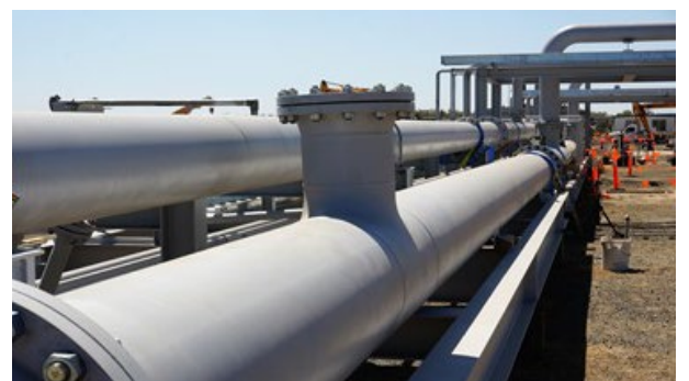
Roma North pipe rack installed
