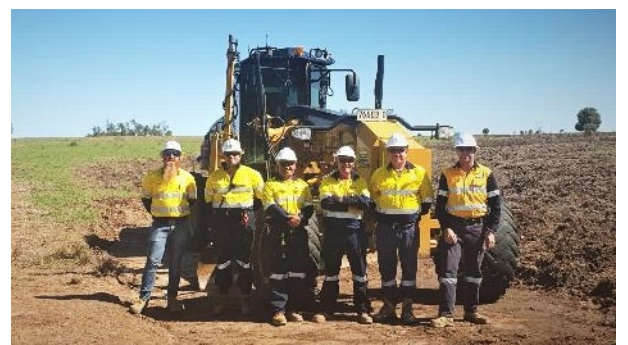
Civil work commences at Project Atlas
