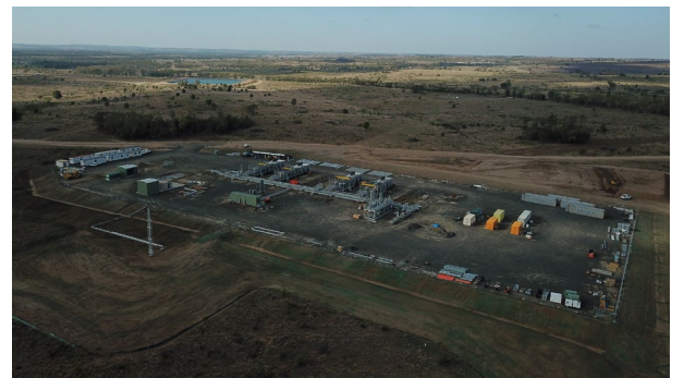
Construction progress at Roma North gas processing facility
