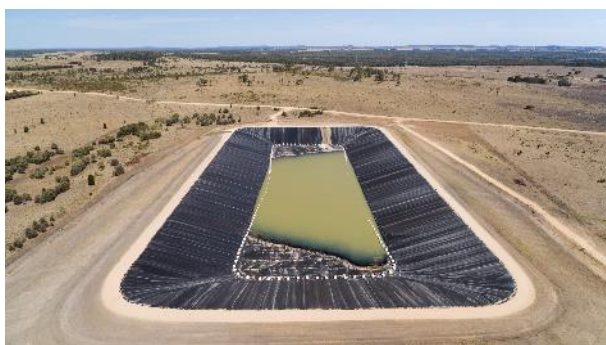
Roma North dam ready for processing facility start-up
