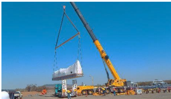
Roma North compressors lifted into place
